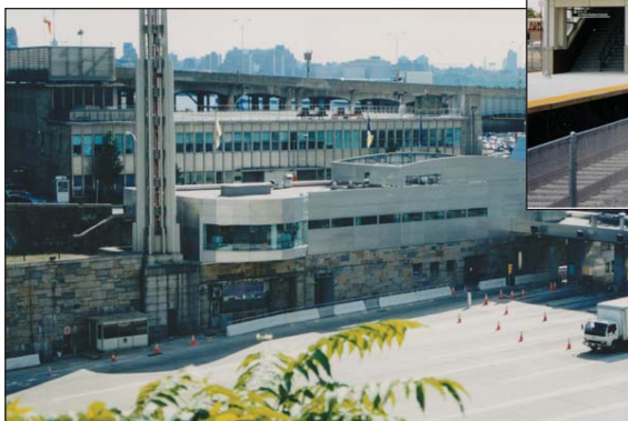
PANYNJ - Lincoln Tunnel Toll Building Expansion
