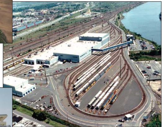
PATH Harrison Yard - Harrison, NJ
