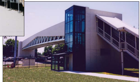
Hofstra University Pedestrian Bridge - Uniondale, NY
