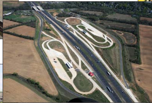
NJDOT - Route 78 Truck Weigh and Inspection Stations
