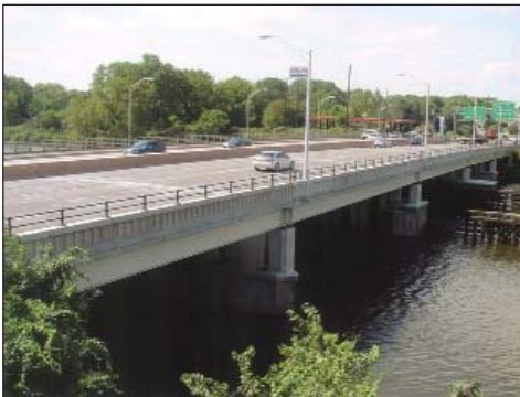
Route 46 over Overpeck Creek Ridgely Park, NJ
