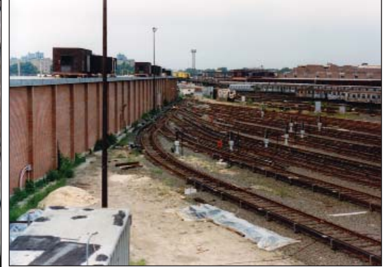
New York City Transit Authority - Coney Island Yard
