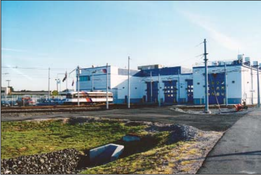
Newark City Subway Rail Maintenance Facility Bloomfield, NJ
