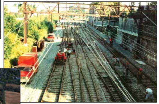
SEPTA Mainline - Track & Bridge Rehabilitation
